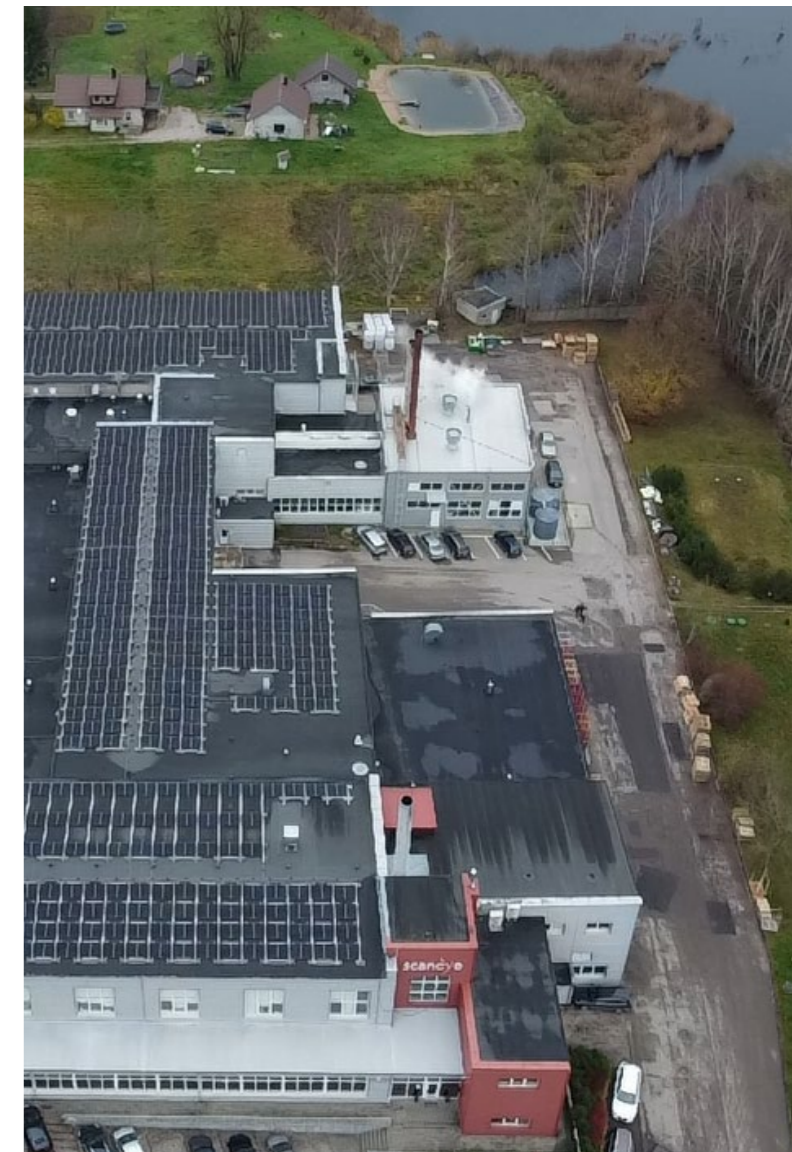
Gabriel's part-owned dyehouse, Scandye, has a solar power system with an estimated annual production of 702 MWh. In the beginning of 2023/24, the capacity will be further expanded with the installation of a new solar power system.
